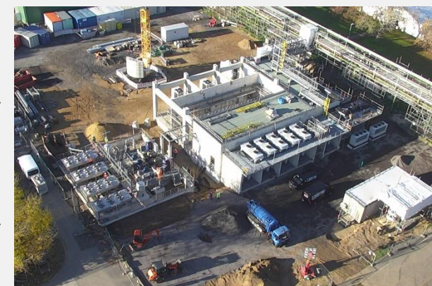
A 10 MW RefHyne electrolyser construction to be completed in mid-2021, Germany
